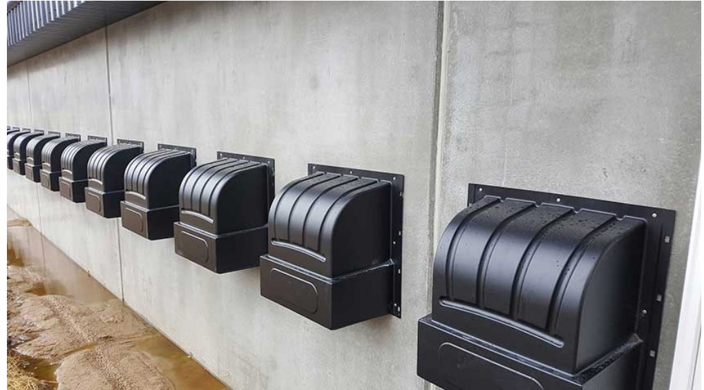
TPI Windhood produced in 90% use of recycled plastics (regrind) – 10% virgin plastics are needed for UV protection
