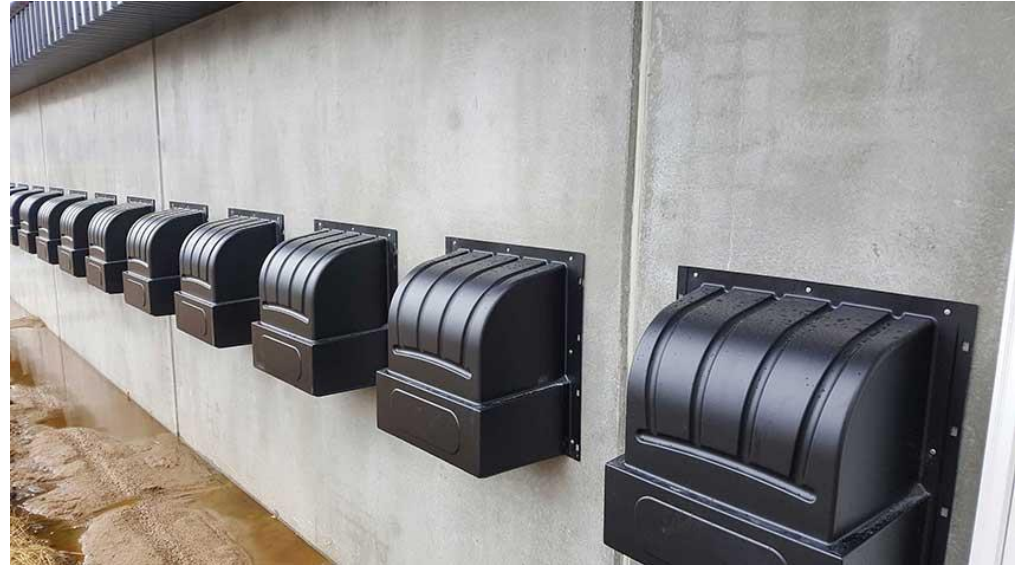
TPI Windhood produced in 90% recycled plastics (regrind) – 10% virgin plastics are needed for UV protection
