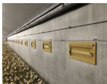
TPI ventilation in a poultry house
